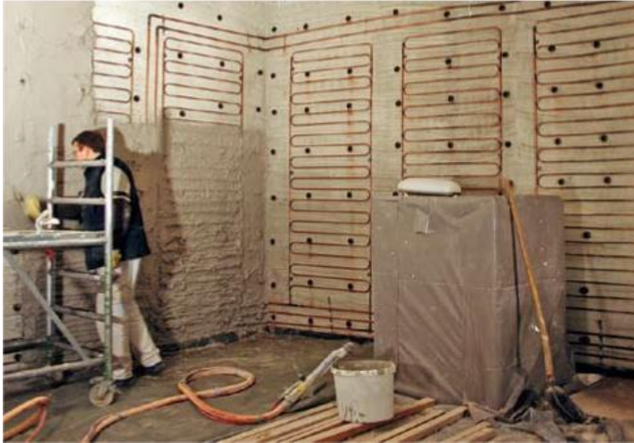
Figure 3.1: Installation of a Hypoplan wall heating system (from: [12])
